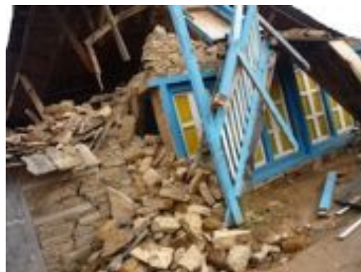
Damage in Pattale 2015 (NAFA)
