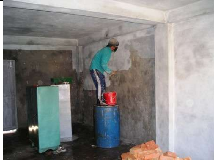
First coat of paint to seal the walls of the clinic
