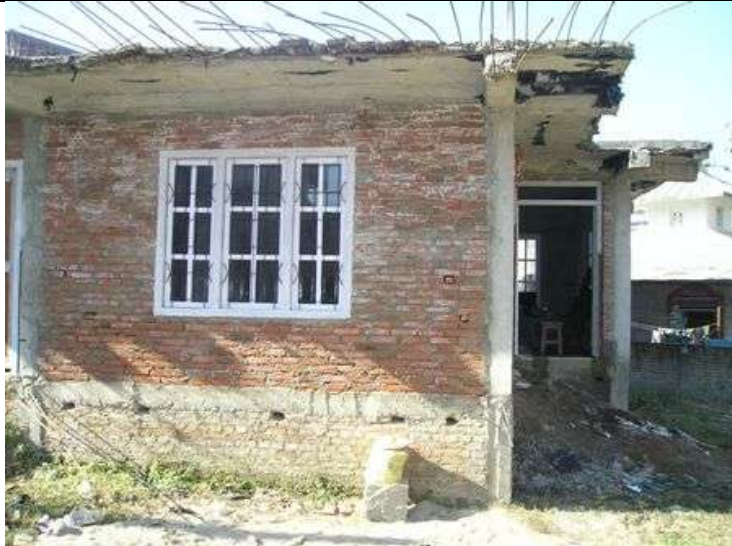
The Red Cross building has three rooms almost completed
